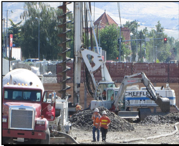
A continuous flight auger (in background) was being used to drill shafts for the bottom seal for the Lincoln Avenue underpass and to fill the shafts with concrete.
