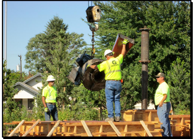
A crew from Granite Construction Company uses a crane to install an old compressor from the former Boise Cascade mill in the center of the Fair Avenue roundabout in June.
