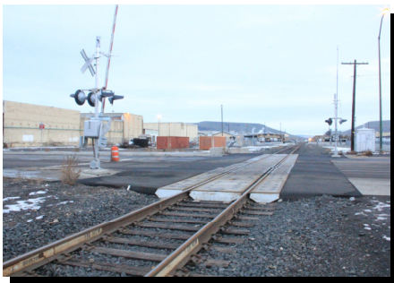
Trains will eventually cross a new bridge above MLK, Jr. Blvd.
